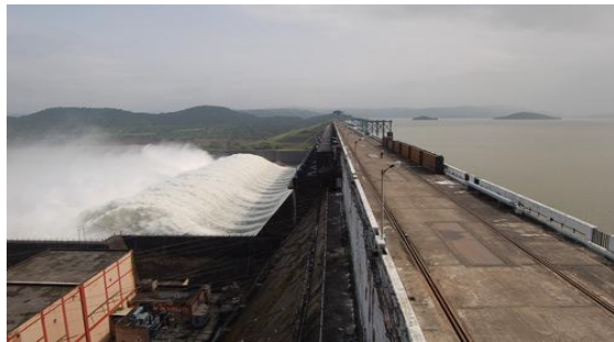
Fig.2. Ukai Dam on Tapi River
